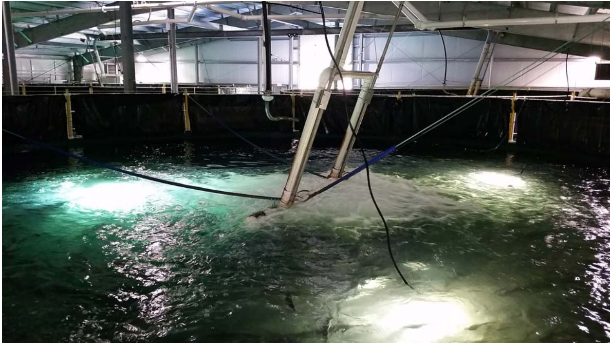
In-tank aeration device
