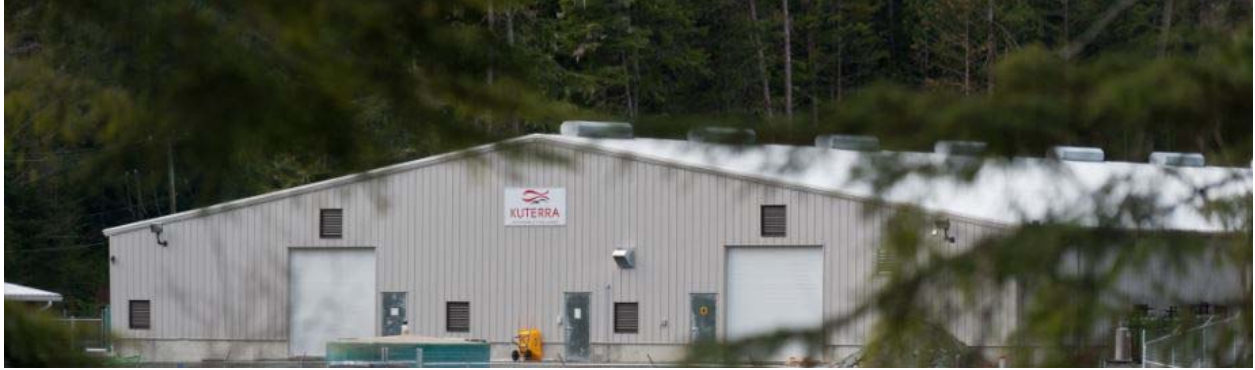
The Kuterra land-based recirculating aquaculture system Atlantic salmon fish farm.
