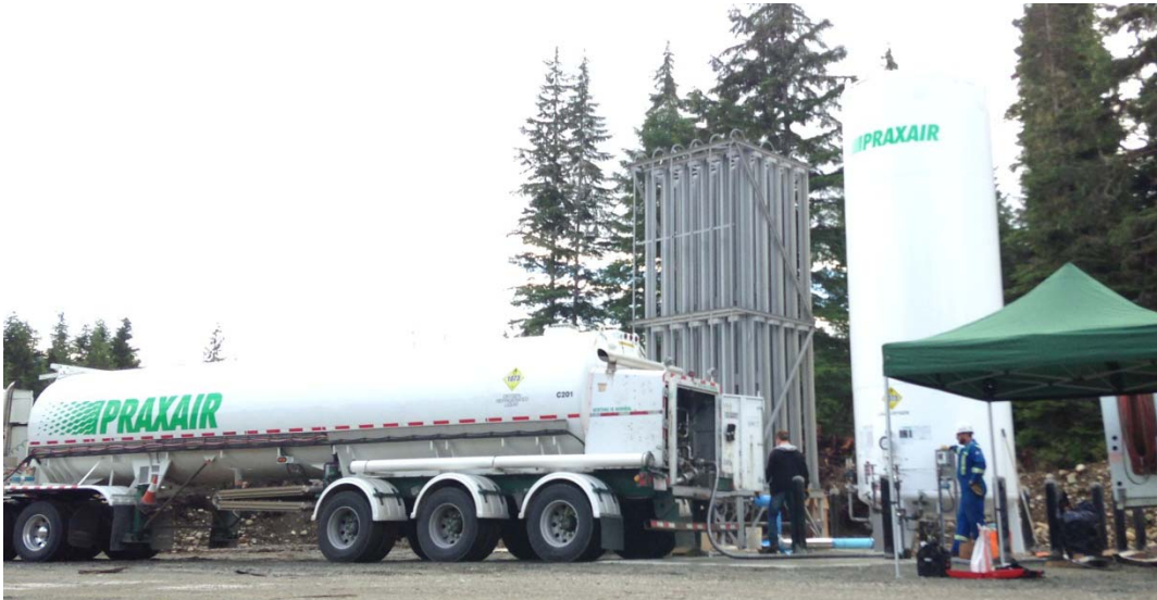
Liquid Oxygen Tank
