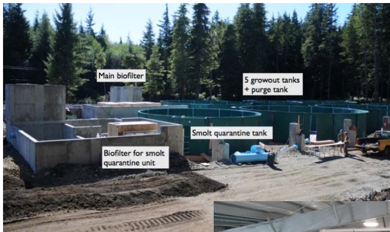
<Biofilters and tanks during construction.
